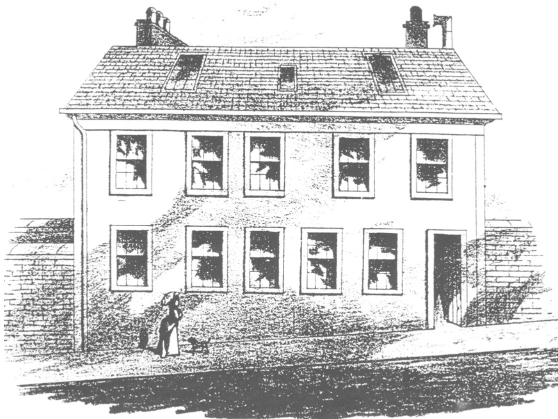
COMMERCIAL SCHOOL, MEETING HOUSE LANE. Erected 1781.
