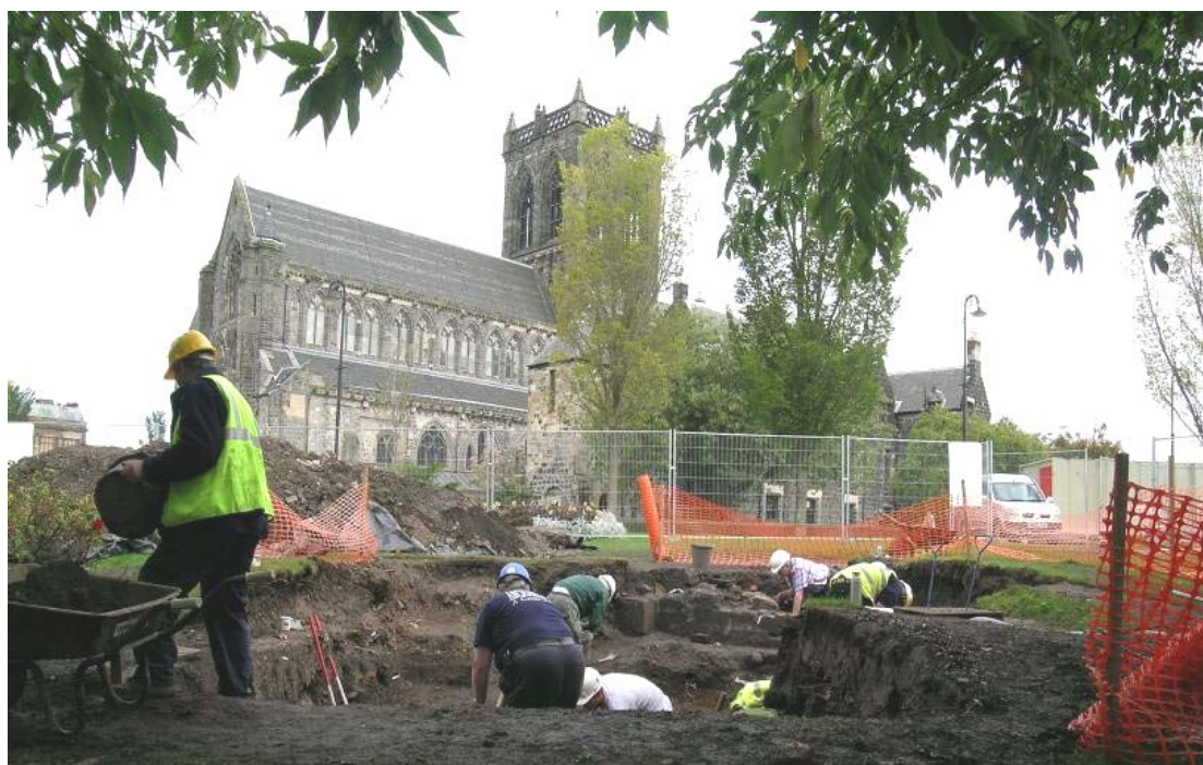
Figure 15: Abbey Drain Dig in progress, Paisley Abbey in background (Bob Will, GUARD)
