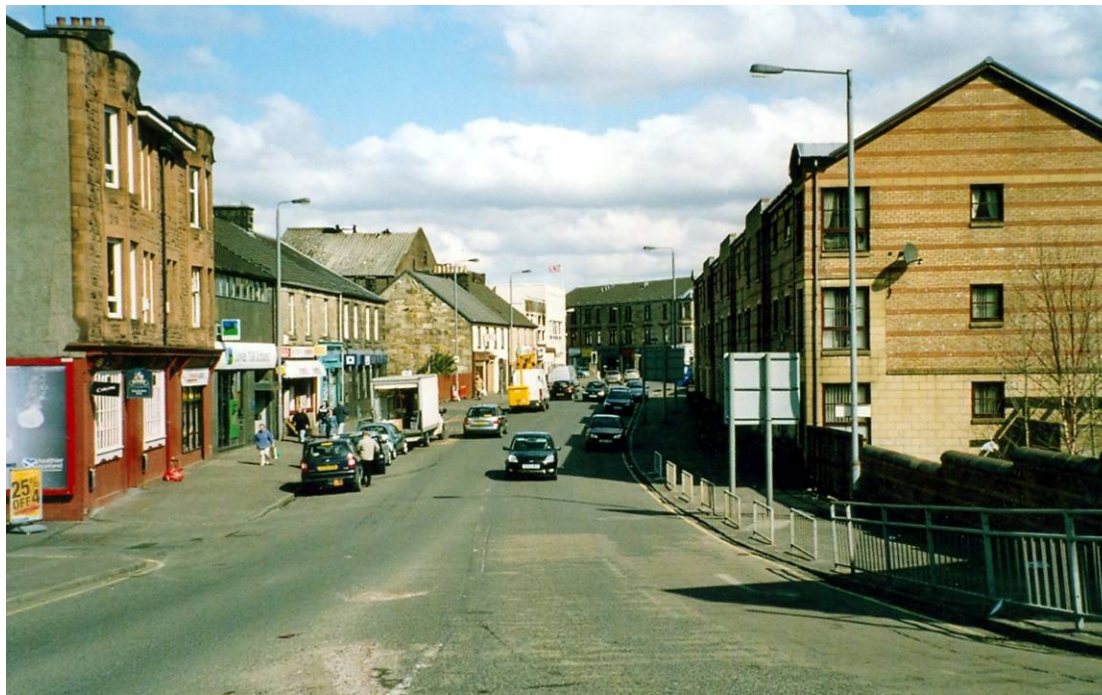
Figure 7: Cross Arthurlie Street, Barrhead (before and after removal of Railway Bridge)
